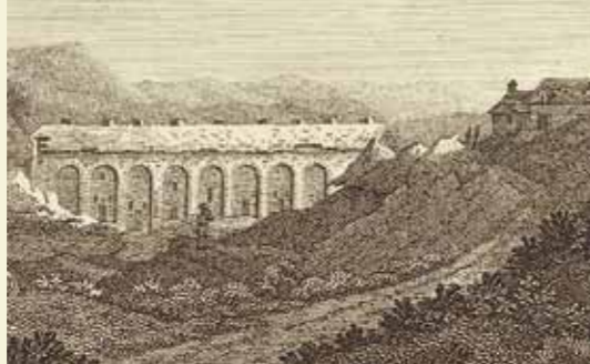
Engraving by Sir Richard Colt Hoare of the 'covered bridge' 1800
