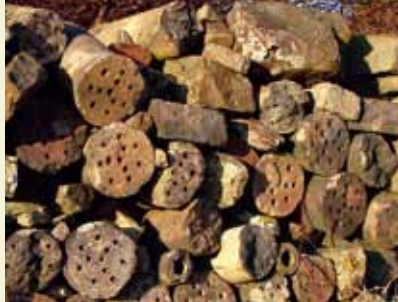
Wall built with Bessemer 'Tuyeres' at Bunkers Hill
