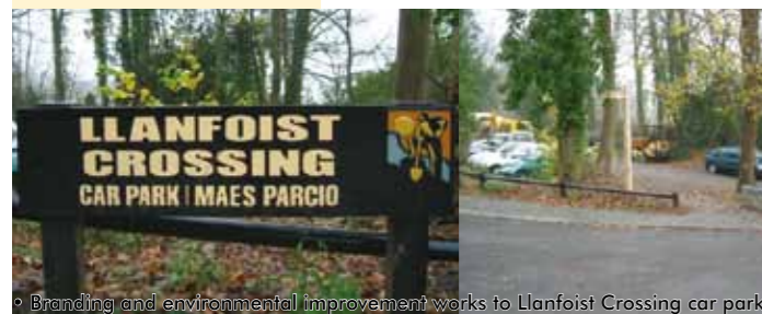
Branding and environmental improvement works to Llanfoist Crossing car park
